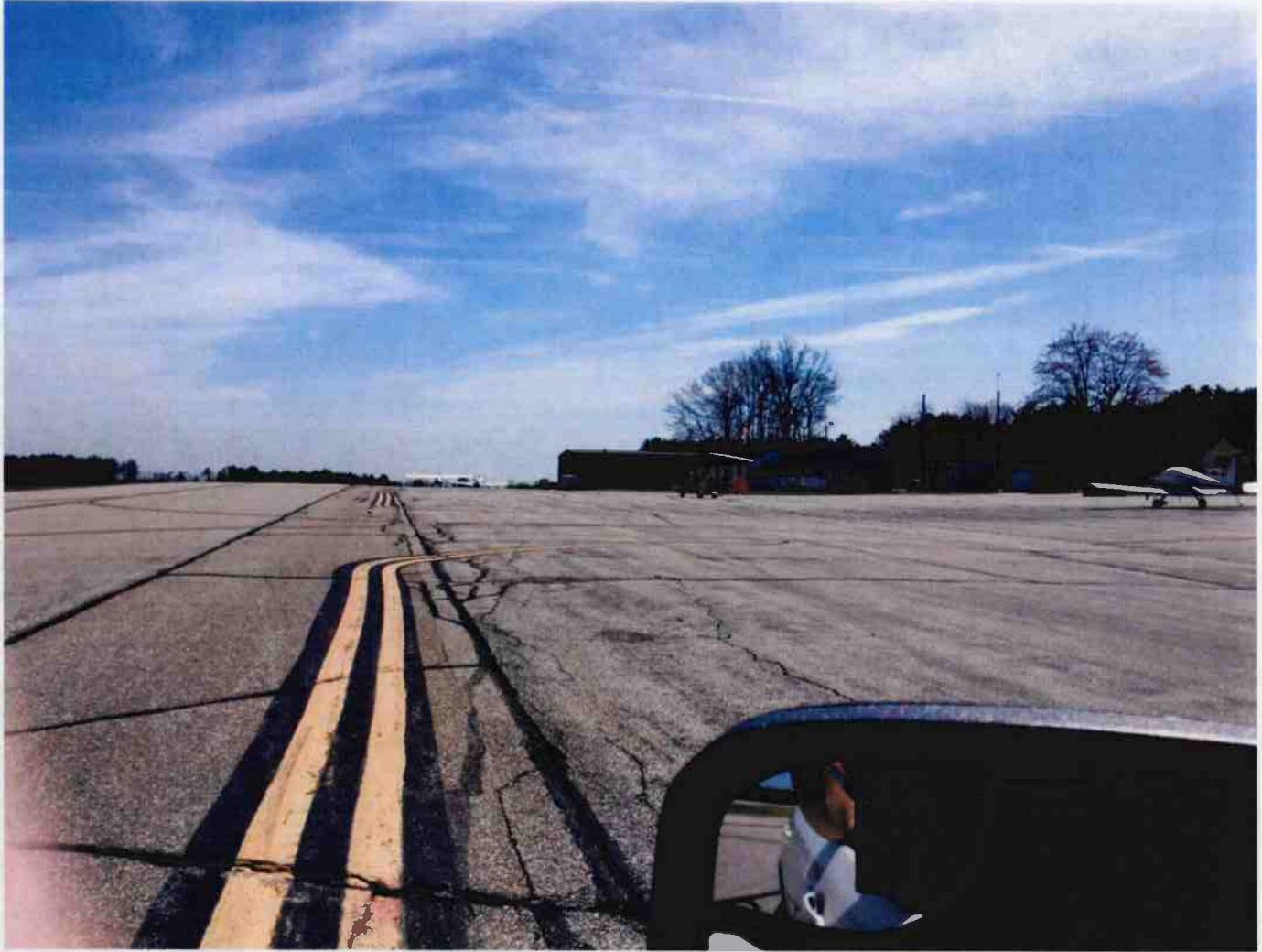
The parking apron near the aircraft hangars is in good condition.
